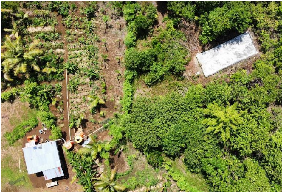
Figure K showing how the Water pan feeds the water tanks. The roof of the Garden house is also plumbed to the Tanks
