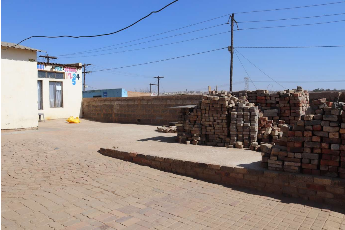
Photo: Letladi Preschool, before finalizing the refurbishment.
